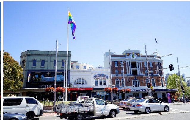
View looking west from Flinders Street
