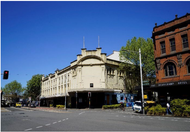
View looking south-east of the Former Olympia Theatre
