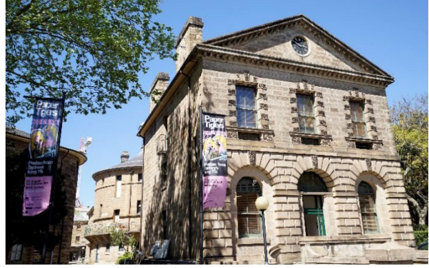
View looking south-east of the NAS (former Gaol) from Forbes Street
