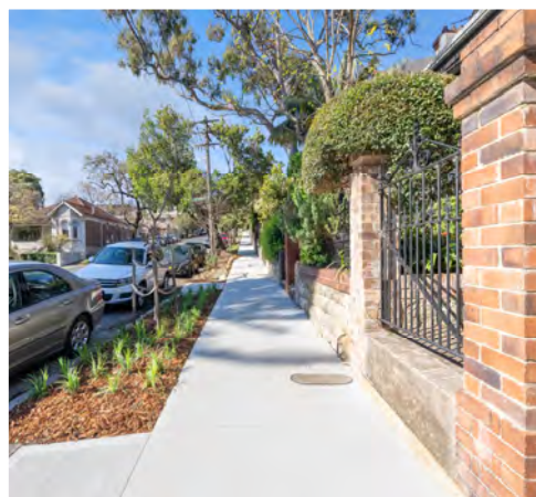
Images: Eglinton Road, Glebe Footway Renewal Works 2021
