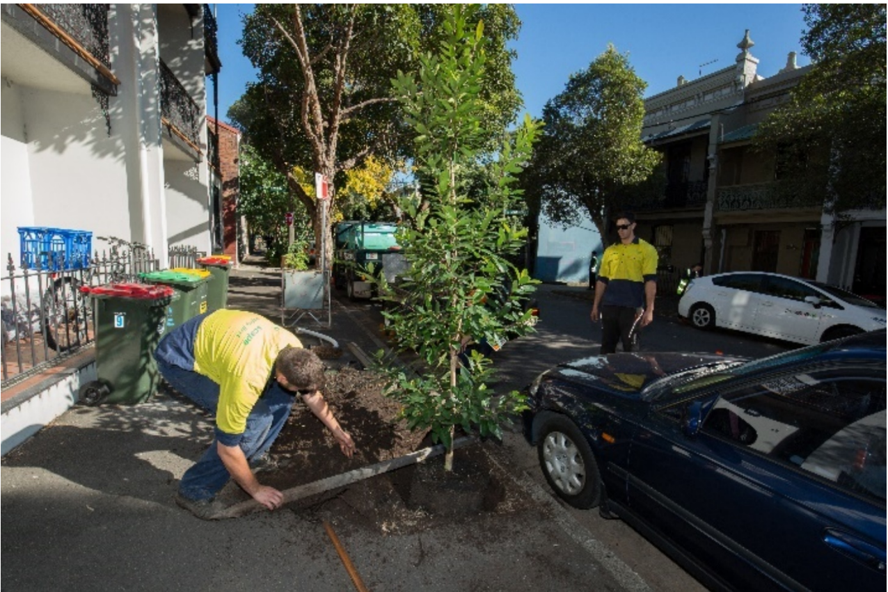
Tree roots being pruned prior to planting and ensuring correct placement in the tree pit. City of Sydney 2016.
