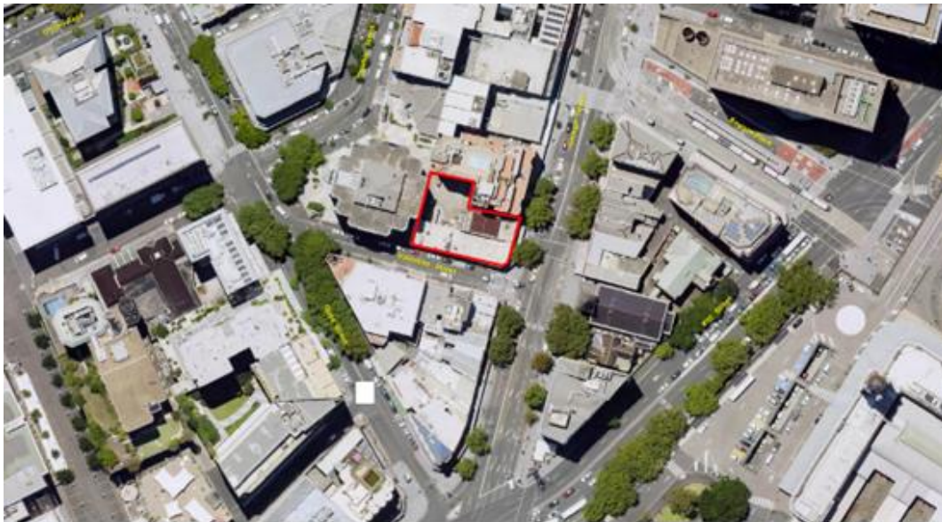
Figure 1: Aerial image of subject site (in red) and immediate vicinity
