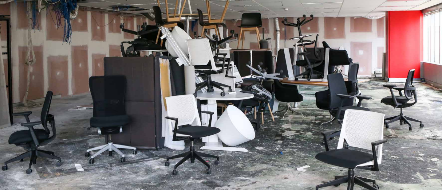
Office stripout waste from 580 George Street, Sydney / Image: Katherine Griffiths
