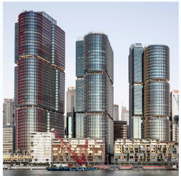
Barangaroo South Precinct / Source: Lendlease
