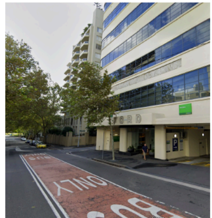
Riley Street, looking northeast towards Ford building
