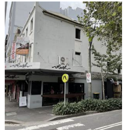
Subject Site 238-240 Reservoir Street
