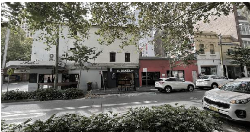
Subject Site 238-240 Reservoir Street
