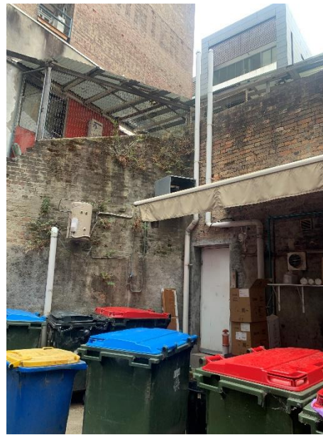
Figure 22 – Rear dock/service yard accessible via Foster Lane.
