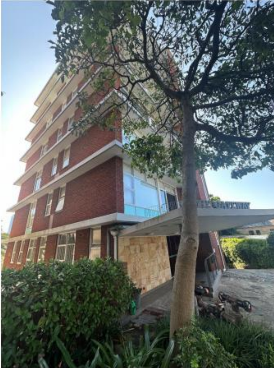
Figure 4. Gateway, 3 Wylde Street. Source. GML Heritage, 2024.
