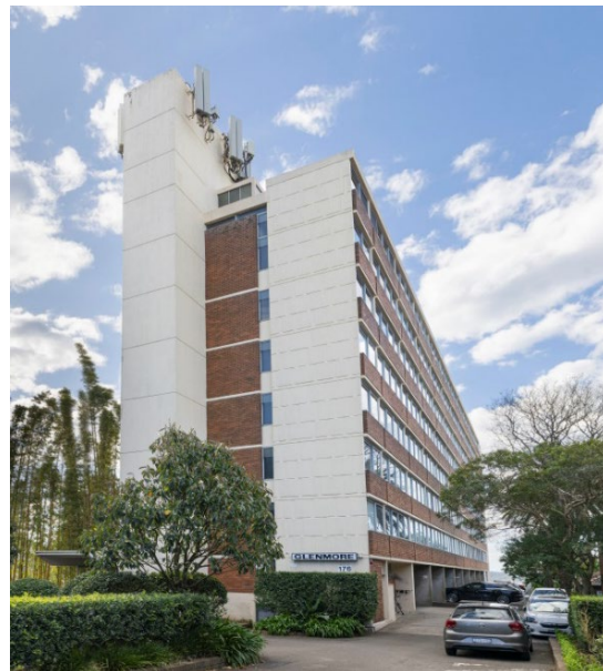
Figure 2 Glenmore Apartments, 176 Glenmore Road, Paddington, 1966, a slab block with extensive views to the harbour. Designed by HP Oser Fombertaux & Assoc Architects. (Source: realestate.com.au)
