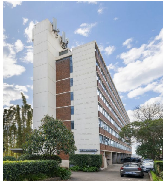
Figure 2 Glenmore Apartments, 176 Glenmore Road, Paddington, 1966, a slab block with extensive views to the harbour. Designed by HP Oser Fombertaux & Assoc Architects. (Source: realestate.com.au)
