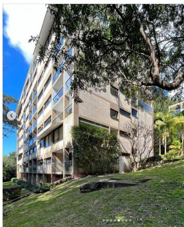
Figure 2 Village Towers (Arlington), Edgecliff (1965–1966), is a significant example of Seidler's evolving use of planning and construction prototypes first applied in Ithaca Gardens. (Source: Philip Thalís)
