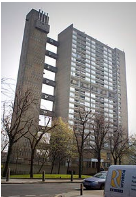
Figure 1 Balfour Tower, Poplar, a Grade II* listed tower block designed by Erno Goldfinger in 1963 for the London County Council, built 1965–1967, which adopts the same separated circulation tower as Aquarius. (Source: Wikimedia)
