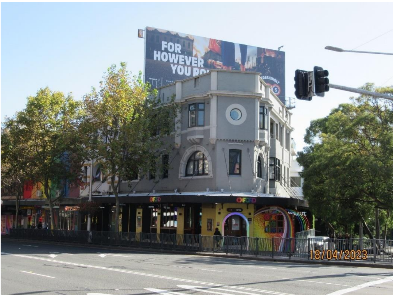
Figure 2. Oxford Hotel at 134 Oxford Street, Darlinghurst
