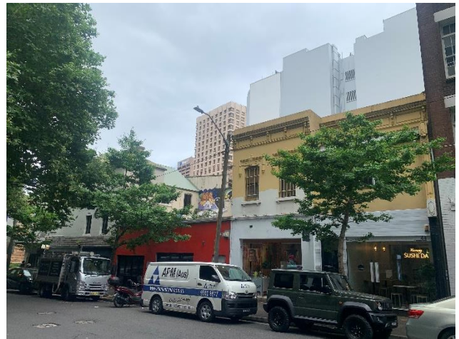
Figure 6 – View of secondary façades on Reservoir Street
