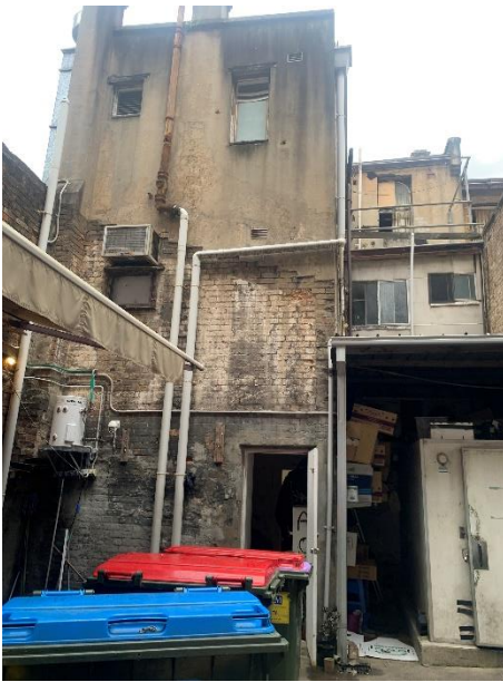
Figure 21 – Rear dock/service yard accessible via Foster Lane.
