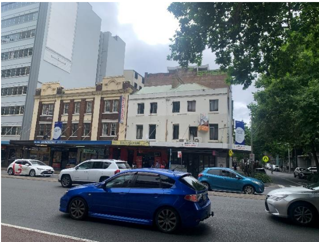
Figure 5 – View of primary façade on Elizabeth Street
