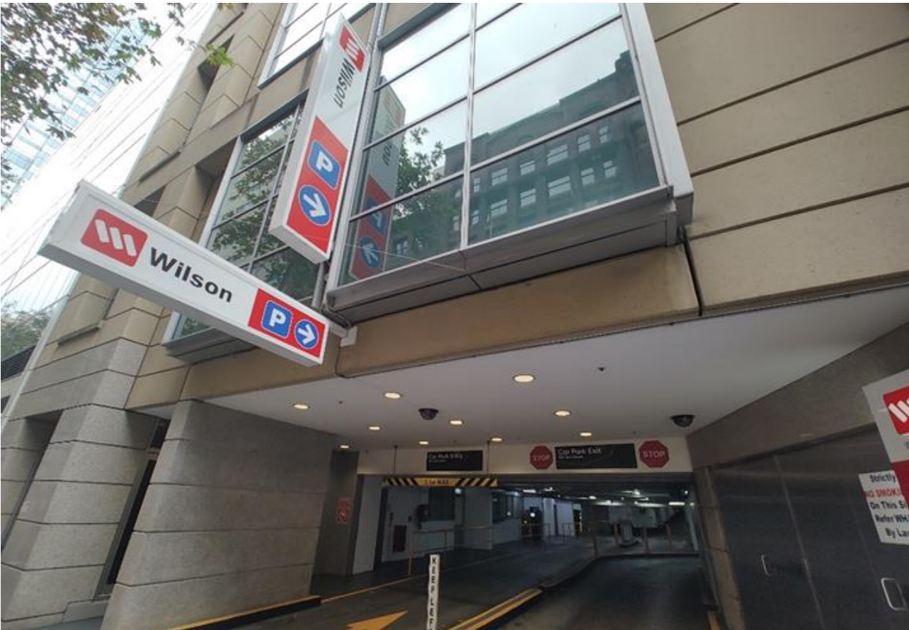
Figure 19 – Front lobby and small retail tenancy at ground-floor level of subject building, at Kent Street Source: Urbis, March 2023
